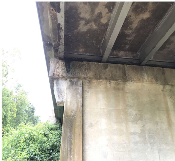
PHOTO 1 Description Bent #3 cap left behind side spalling and delaminated areas.
