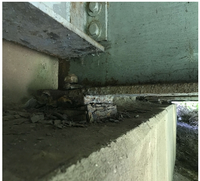
PHOTO 2 Description Typical condition state of flaking rust to bearings due to leakage through joints.
