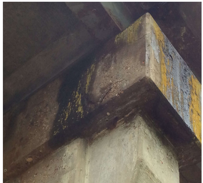
PHOTO 2 Description Deterioration of right end of bent #2 cap
