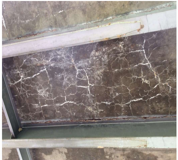
PHOTO 2 Description Efflorescence cracking with leakage between girders #3,#4 in deck soffit.
