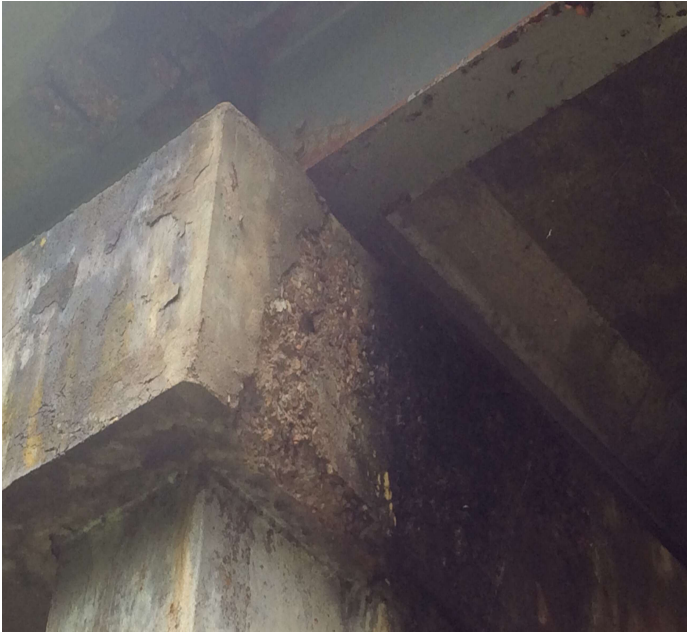
PHOTO 3 Description Deterioration to left end of bent #3 cap
