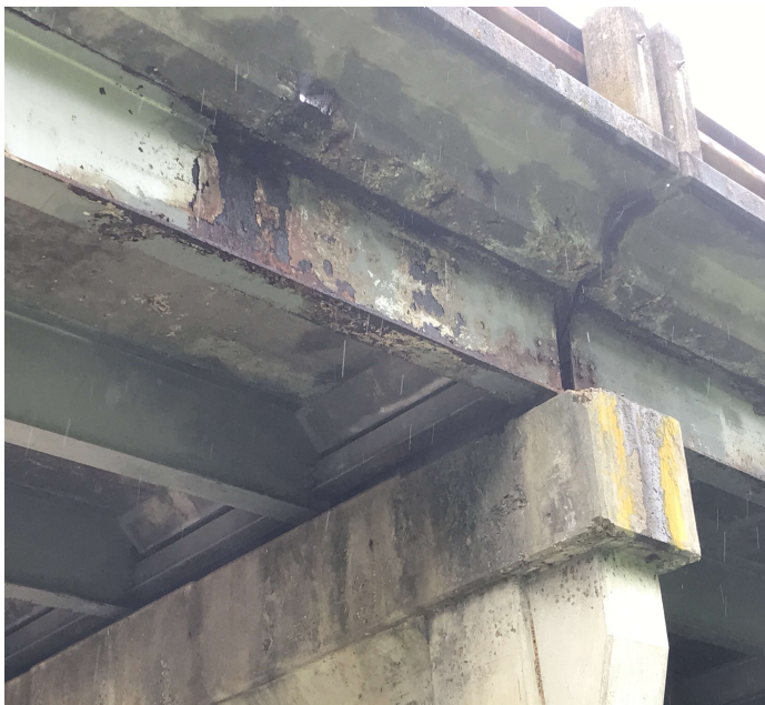
PHOTO 1 Description Span #3 girder #5 typical end of girder corrosion
