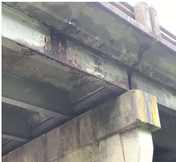
PHOTO 8 Description Span #3 girder #5 typical end of girder corrosion
