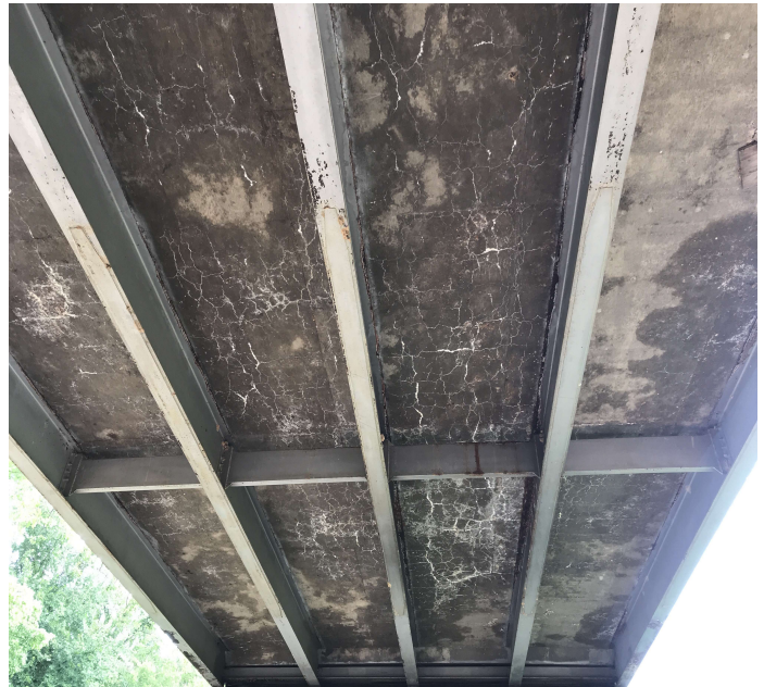
PHOTO 6 Description View of span #3 efflorescence.
