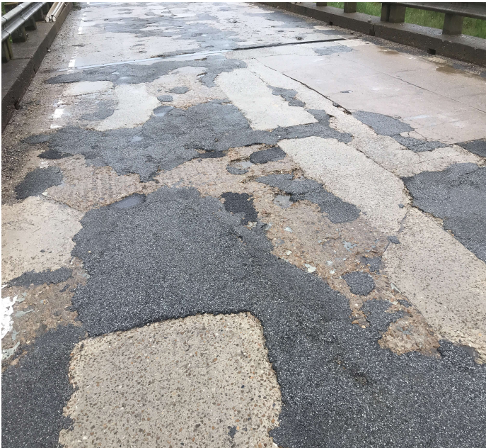
PHOTO 4 Description Span #3 typical spalled patched areas.
